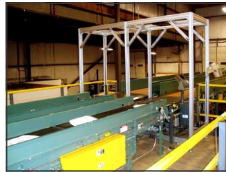
New Conveyor and Scales
