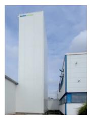
To increase the existing facility capacity, a Kardex Remstar Shuttle XP VLM can be installed outside the building and walled in with pass-through access.
