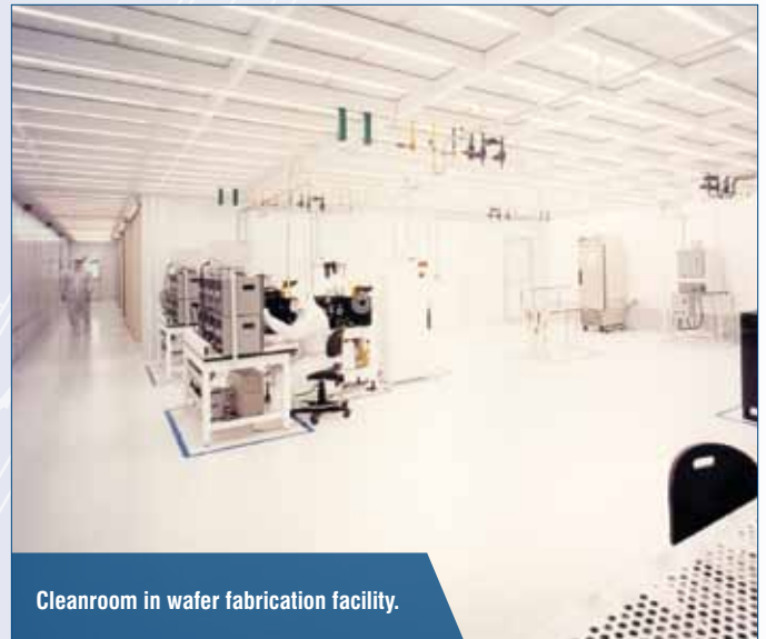
Chase side of a bay and chase cleanroom featuring piping, conduit, and support equipment.
