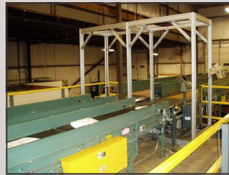
New Conveyor and Scales
